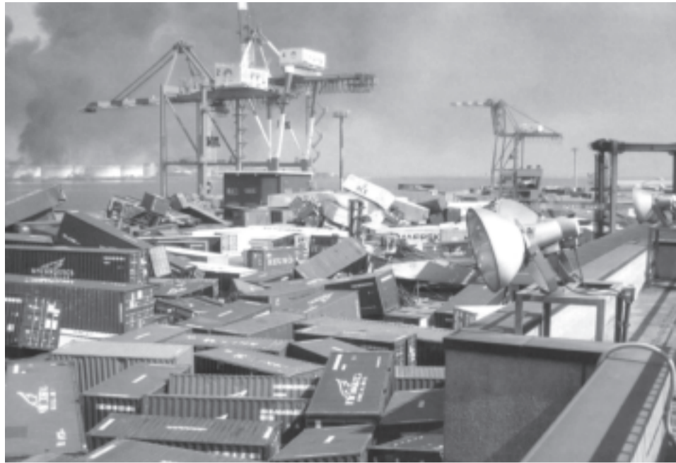
The destruction of the container yard at the Sendai-Shiogama Port shows the extent of the damage caused by the March 11 earthquake and tsunami which hit the North-East regions of Japan.
